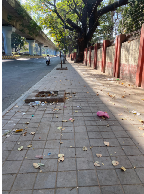
1.0: A clean street, except for a few pieces of litter.
